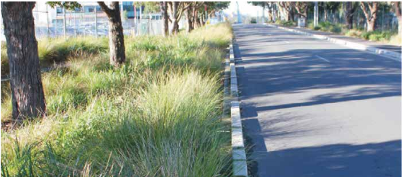
FIGURE 42: Raingarden at Murray-Rose Avenue in Sydney Olympic Park. The sloping road surface allows draining stormwater straight into the vegetated area on the left side. Open curb stones allow water flow whilst holding back larger debris. Image © S. Pfautsch.
