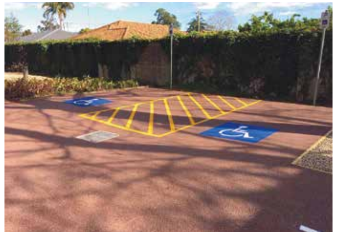
FIGURE 37: Example of recycled rubber mix used in a car park in Penrith, NSW. Image © FiltaPave ( https://filtapave.com.au/ )
