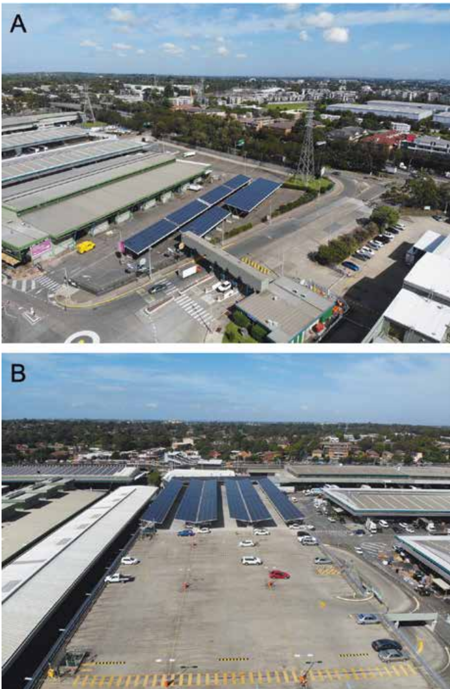
FIGURE 21: The solar car parks at the Sydney Markets. (A) Car park A was covered with asphalt and it was located between the main entrance and the flower market. (B) Car park B had a concrete surface and it was located at the top of a multi-storey parking lot. Image © S. Pfautsch
