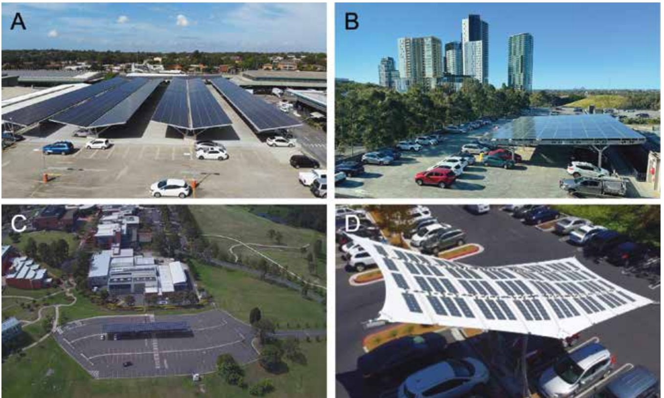
FIGURE 34: Examples of solar shade structures over car parks. A: Sydney Markets in Flemington. Image © S. Pfautsch. B: Car park P3 at Sydney Olympic Park. Image (c) S. Pfautsch. C: Solar car park at Kingswood campus of the University of Western Sydney. Image (c) S. Pfautsch. D: a combination of shade fabric with photovoltaic panels at Google company (Li and Zanelli, 2021).
